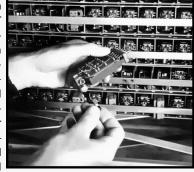
States Air Force. TRADIC contained nearly 800 transistors, which replaced the standard vacuum tube and allowed the machine to operate on fewer than 100 watts, which is onetwentieth of the amount of power required by a comparable vacuum tube computer.
